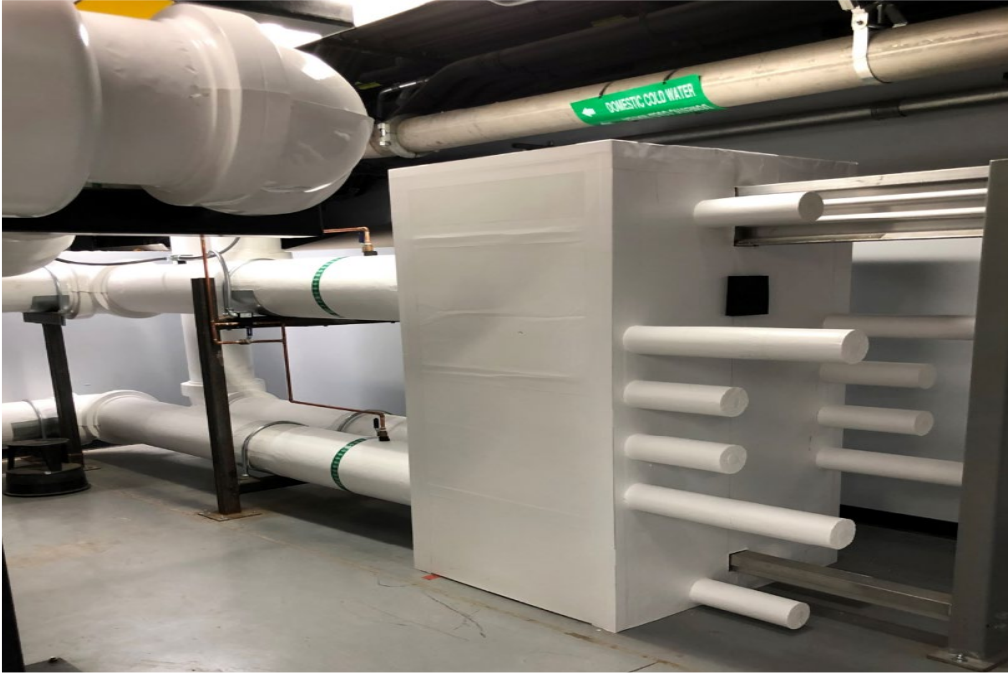
Figure 5 Heat Exchanger installation photo
